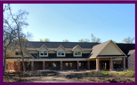
Have you seen the progress of our new Education/School Building? It's looking great!
